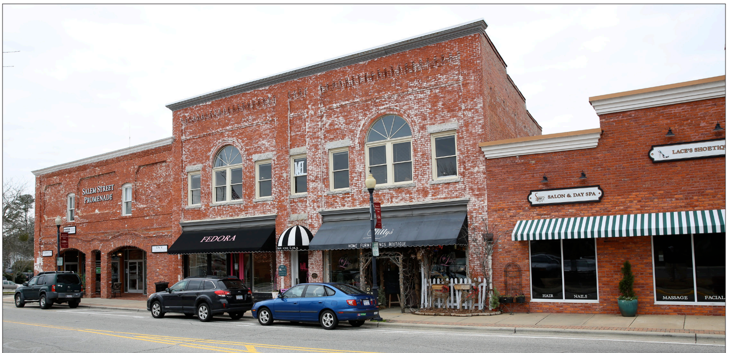
The owner of the restored Hinton & Son Hardware building in downtown Apex (center building) received a 20 percent state Historic Preservation Tax Credit. The owners of the adjacent buildings restored their properties without the tax credit. Cultural Resources Secretary Susan Kluttz featured the Hinton building on her tour to promote the restoration of the expired restoration tax credit. (Carolina Journal photo by Don Carrington)
